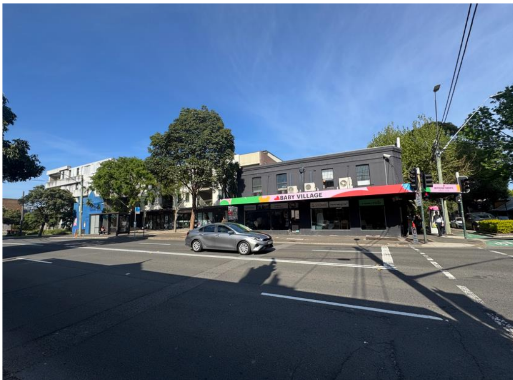
Figure 2: Site viewed from Botany Road facing west
