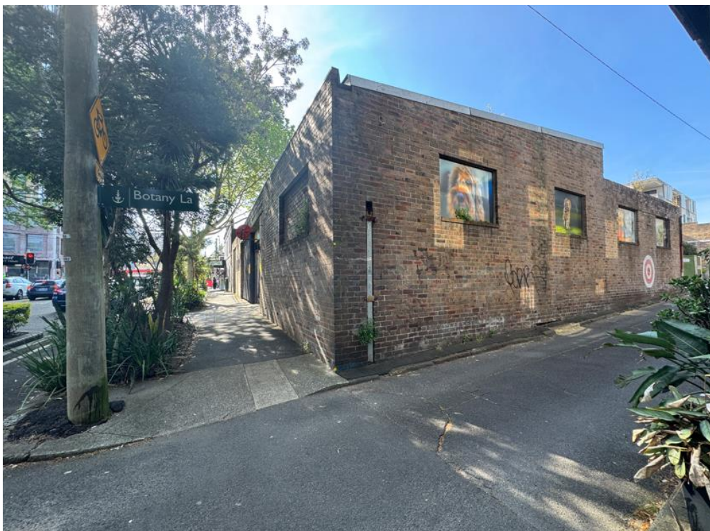
Figure 4: Site viewed from Botany Lane
