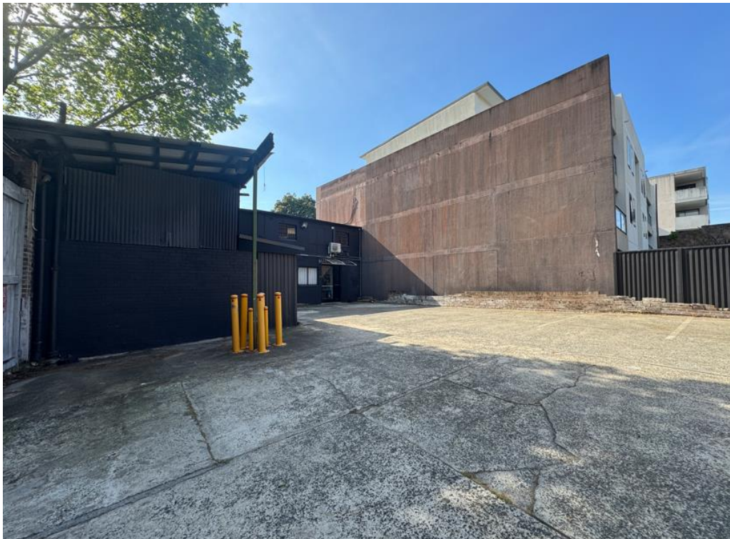
Figure 6: Existing car parking area of the site showing interface with the southern adjoining property at No. 138-142 Botany Road
