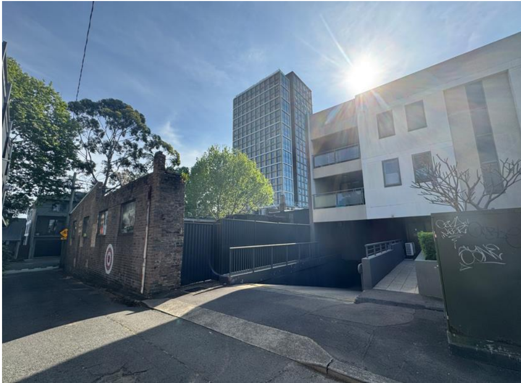
Figure 5: Site rear viewed from Botany Lane
